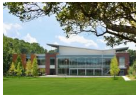
Virginia Wesleyan University's recently completed Greer Environmental Sciences Center
